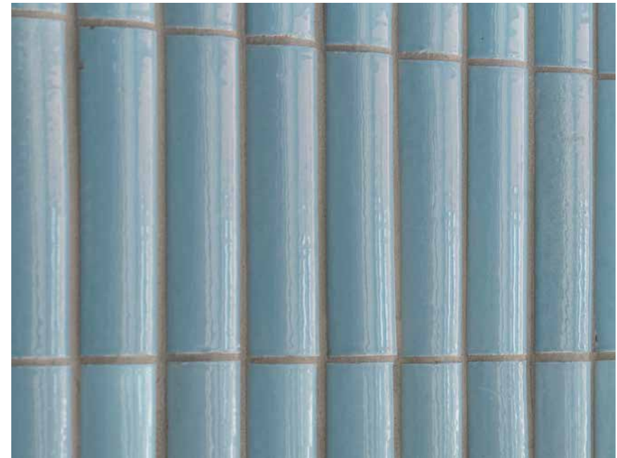
Plaquette convexe bleue, pose verticale à joints filants Blue convex brick slips, laid vertically with continuous joints
