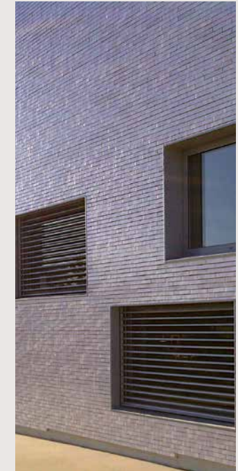
CLADDING BRICKS FOR CAVITY WALLS* Facing bricks for cavity walls also called wall cladding
