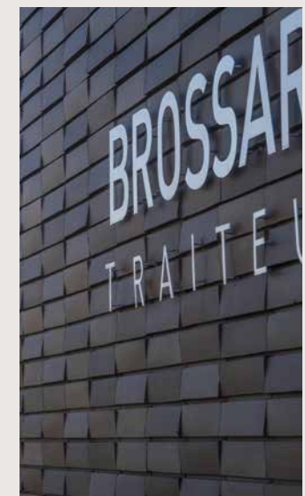
ACROBRIC SMALL SHINGLES* Dry-fitted laying on metal or wooden frameworks and brackets
