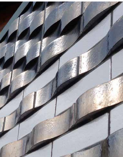
Plaquette hirondelle / Waves brick slip
