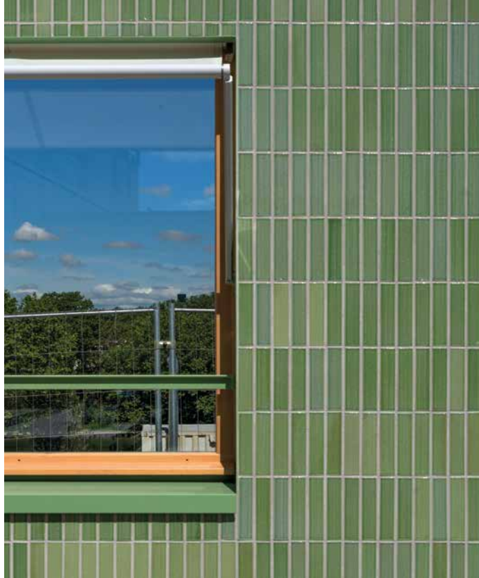
Plaquette verte, pose verticale en 1/3 Green brick slip, laid vertically
